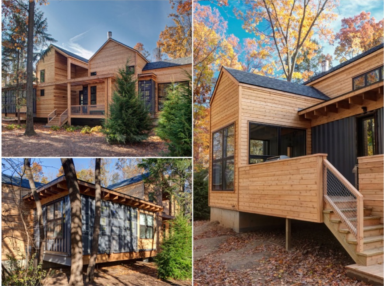
Figure 2: Union Pier, MI home built by Stone's Throw Builders.
