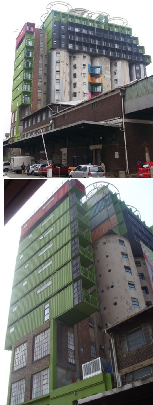
Figure 3: Mill Junction, Johannesburg, South Africa - Citiq, Property Investment & Management Company
