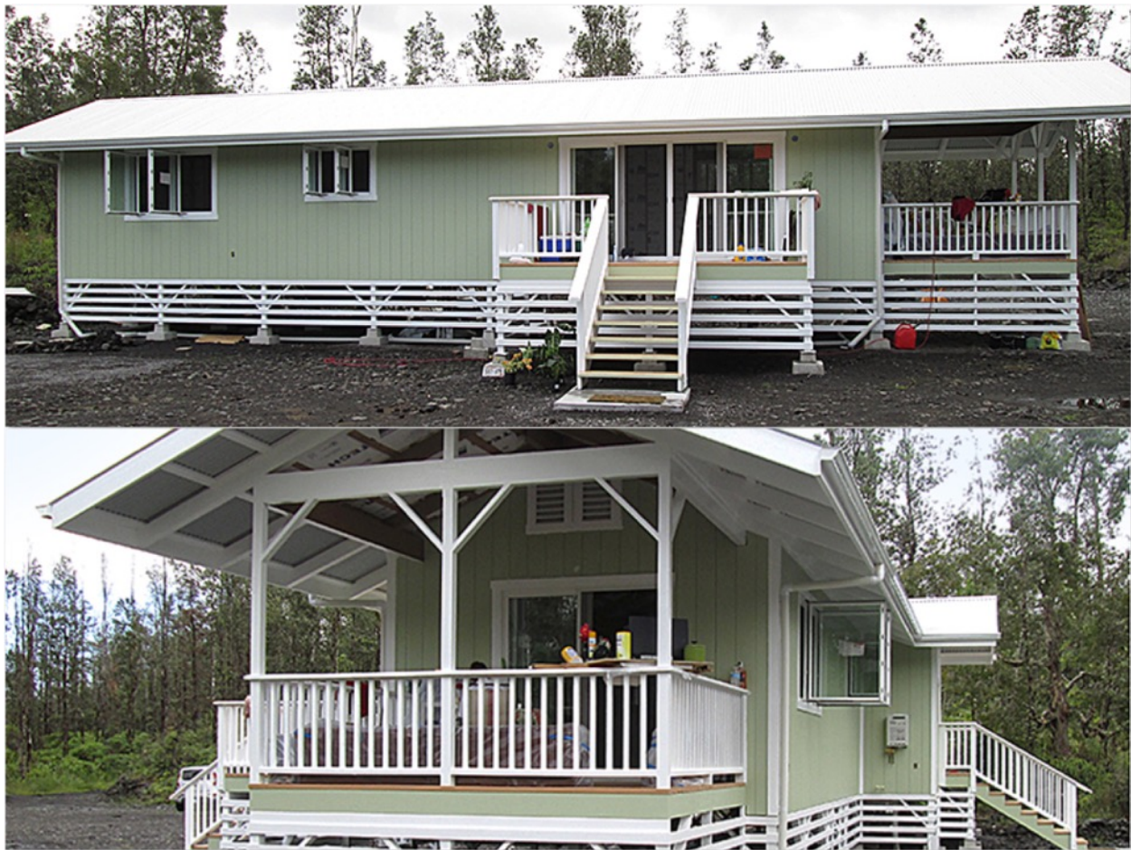
Figure 9: Lava Runner Series - Affordable Portable Housing, Hawai'i - See Floor Plan in Addendum
